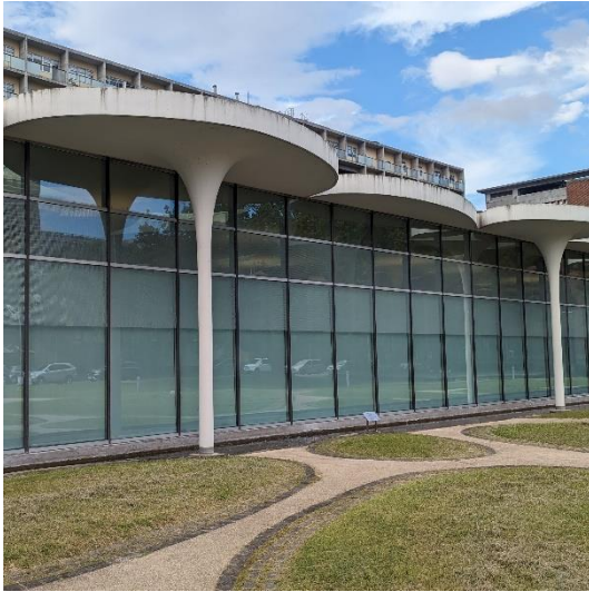
(a) Glass curtain wall
