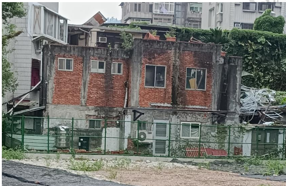
Figure 1-1 Brick wall with openings
