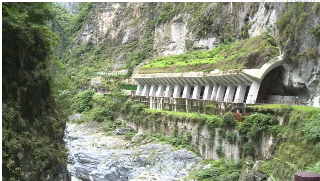
Figure 1-1 Open-cut tunnels with EPS (Expanded Polystyrene) foam covered on top for rockfall protection.
