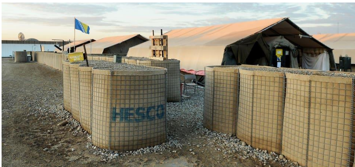
Figure 1-4 Barriers consist of HESCO bastions (Forbes, 2023)
