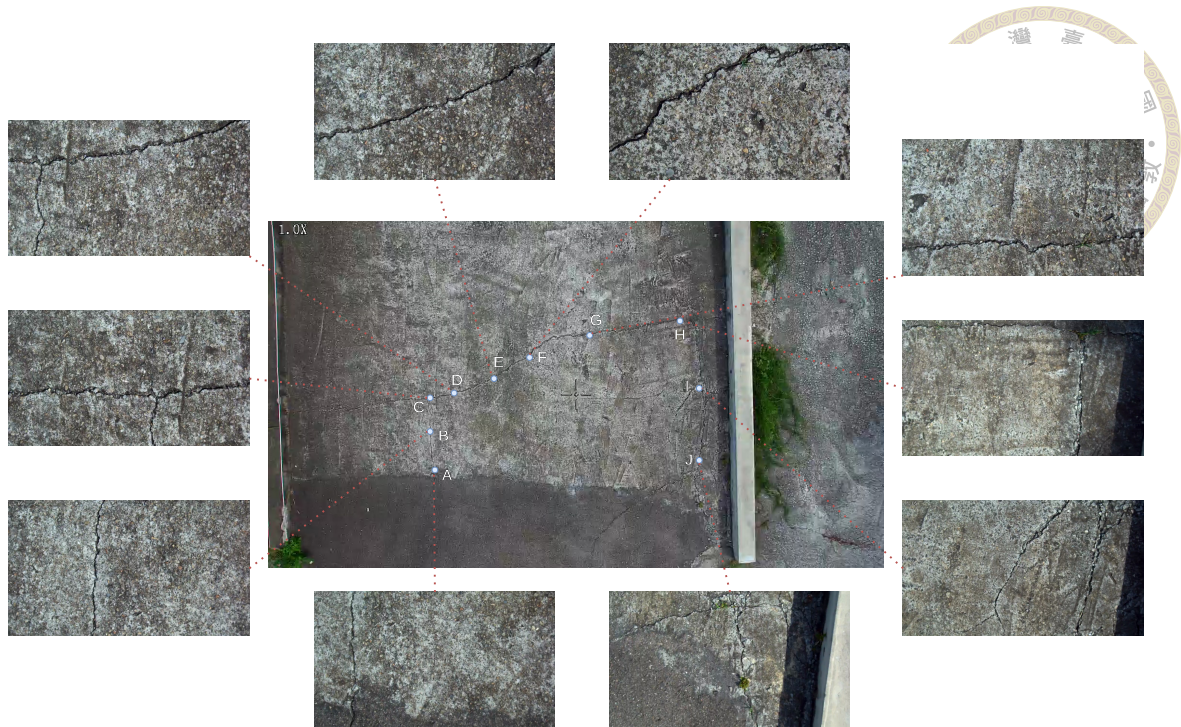
Figure 3.8: The path of an inverted U-shaped crack starts capturing from the bottom-left corner, moving from point A to J, showing each movement trajectory. Using our trained deep reinforcement learning model to determine directions, coupled with the aforementioned constraint to prevent the drone from flying backward, enables automated capturing of the entire inverted U-shaped crack.
