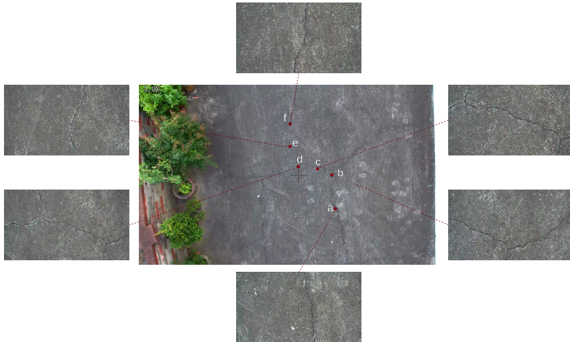
Figure 3.20: The crack pattern in this experiment is characterized by irregular branching. However, due to the preceding setup, the drone is prevented from retracing its path. During the process, crack capture will proceed sequentially from points a to f .
