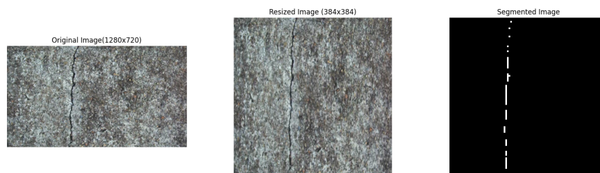
Figure 3.10: At point B, the segmentation results of the detected crack are obtained. After detecting the crack, the segmented image data is fed into DDQN (Double Deep Q-Network) for prediction, followed by forward flight.
