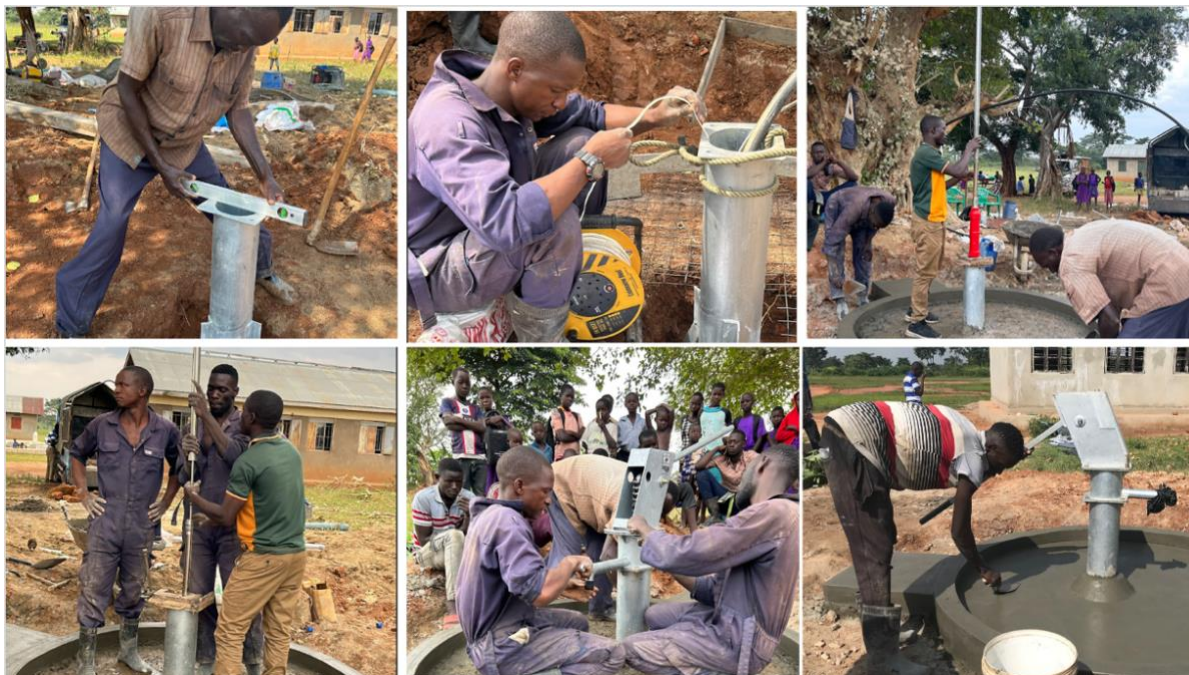
Figure 9: Construction and installation of the borehole (Love Binti International, 2024)
