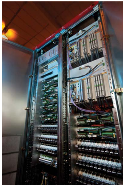
圖 4-3 伺服器層級之儀控設備(Computer-based instrumentation and control systems) (圖片來源: [17])
