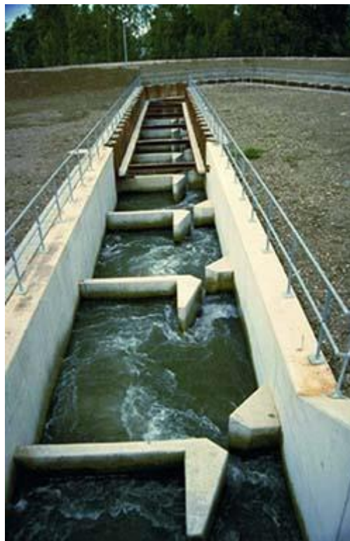
Fig 1.1. Ventrical slot fishway (FAO)
