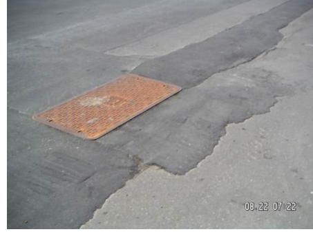
(b) An anomalous pavement and manhole
