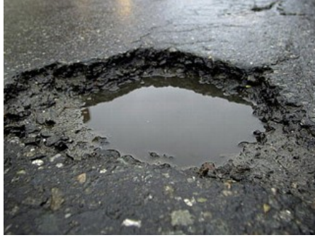
(a) A severe pothole on the road
