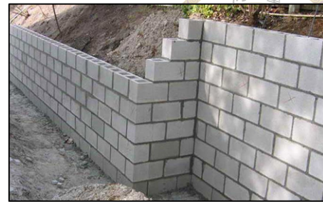
Figure 1.3: Example showing partial completion of construction on the progress reporting date
