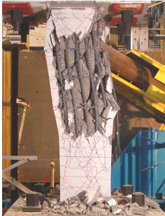
Figure 3-11. Specimen 4NL crack pattern before collapse (6%) (Weng 2007)
