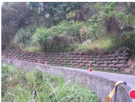
圖 8. 傳統框架工法之擋土牆 Fig.8 The wooden retaining wall constructed by traditional method
