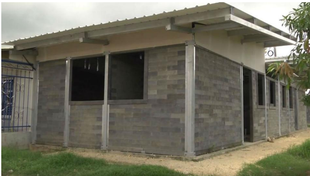
Figure 1. 6 BRICKARP in Colombia as an example of building made from plastic bricks (Source: TRT World)
