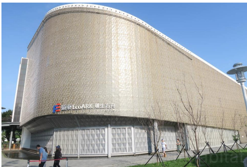
Figure 1. 5 EcoARK in Taipei as an example of building made from plastic bottles
