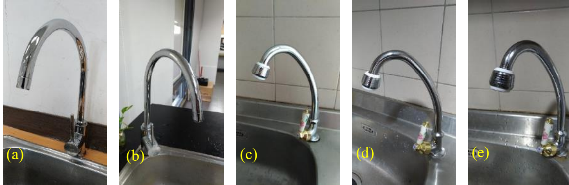
Figure 2. Installation of new faucets. (a) Lead-free faucet 1; (b) Lead-free faucet 2; (c) Brass faucet 1; (d) Brass faucet 2; (e) Brass faucet 3
