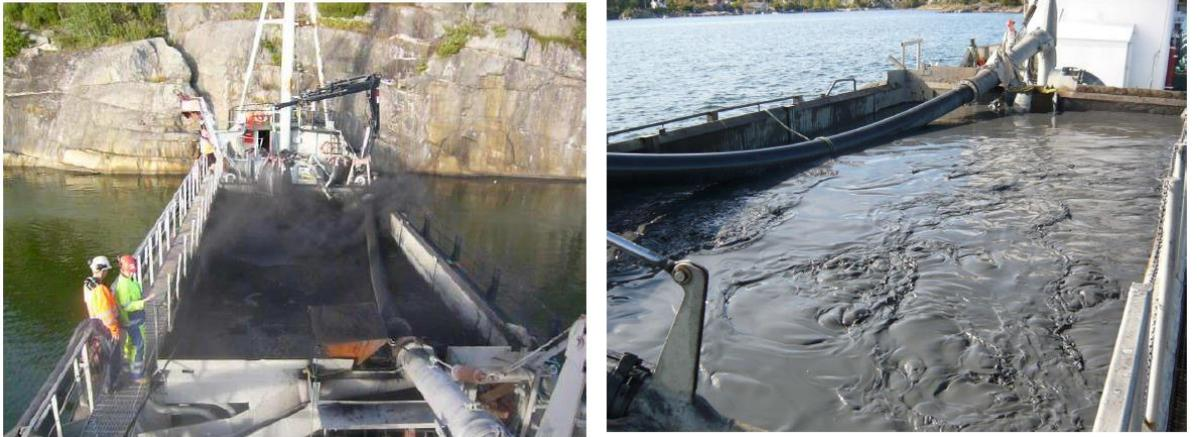
Figure 2-3. Cornelissen et al.[60] premixed AC, clay and seawater and performed a spray thin layer capping by a spraying system on a ship.
