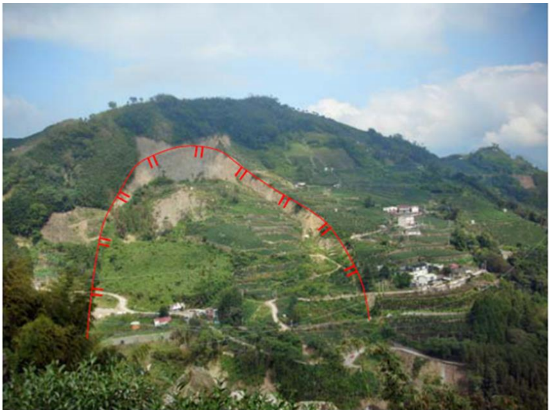
Figure 1-1. The main scarp and lateral scarp are obvious in the photo taken near Yucheliao landslide (Lin et al., 2014). This photo is taken in the direction toward north.
