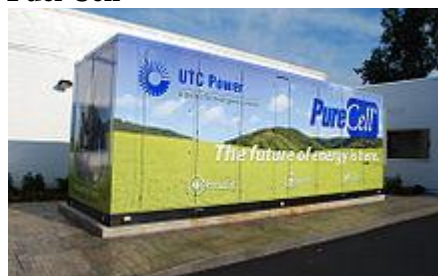
Figure 41: UTC Power 400 kW Fuel Cell
