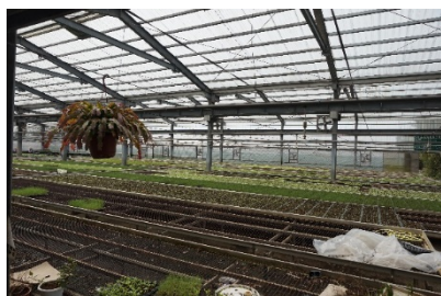
(c) The warehouse taken from section A
