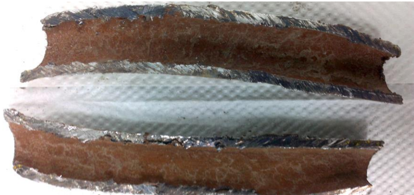
Figure 3 Aged lead pipe which was cut horizontally before experiment
