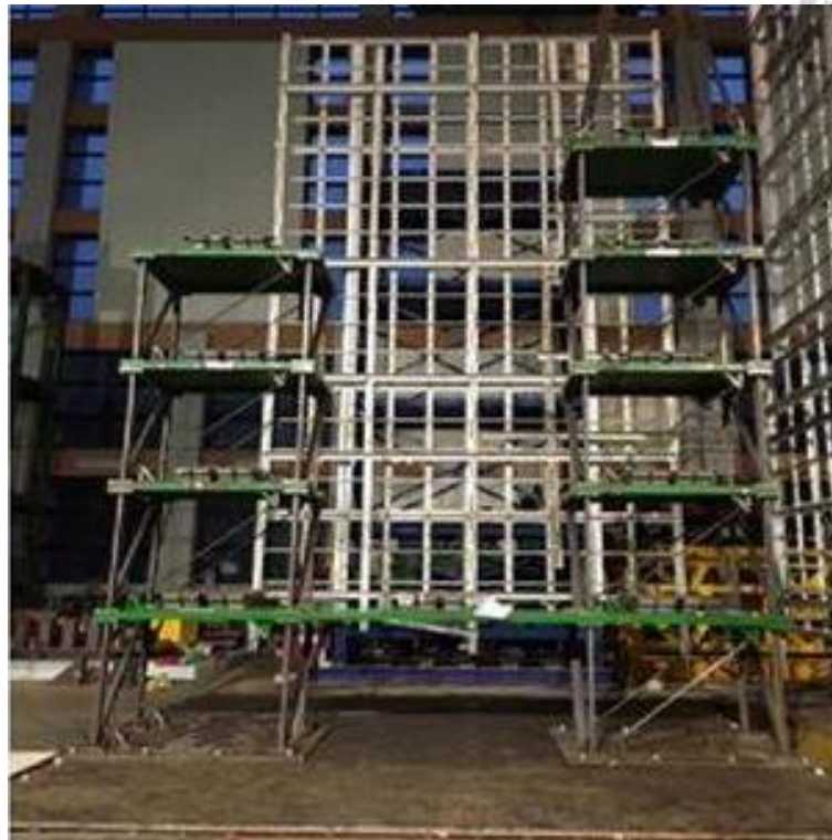
Figure 3-1 The twin-tower steel structure
