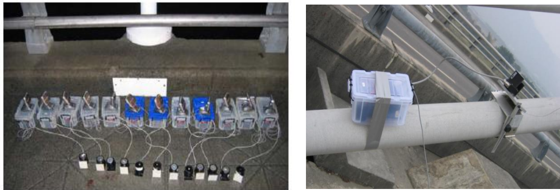
Figure 3.2: pictures of system calibration and cable installation.
